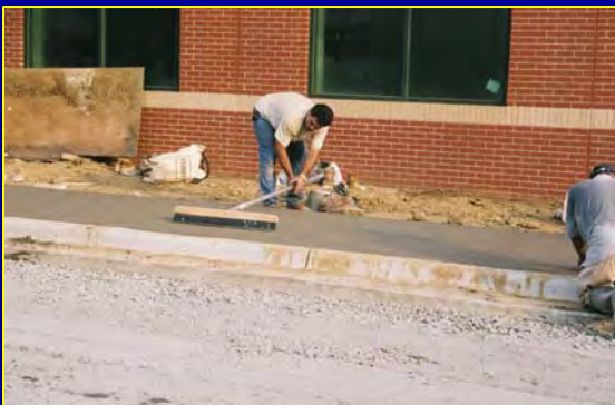
BROOM FINISH AND TOOLING JOINTS
