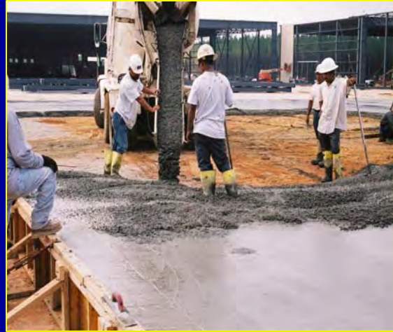
CONCRETE BEING TRUCK DUMPED
