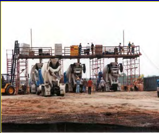
LOADING FIBERS ON PLATFORM
