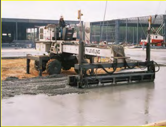
SFRC BEING FINISHED WITH PANS
