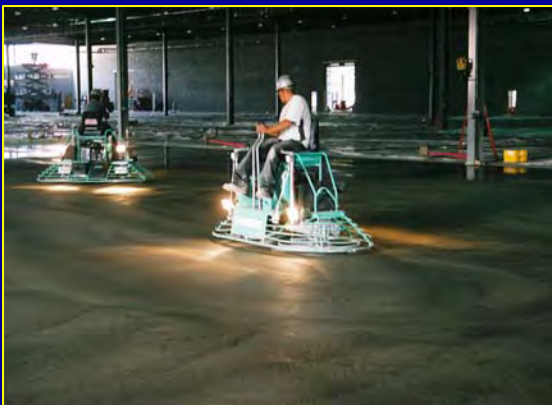
SFRC BEING FINISHED WITH PANS
