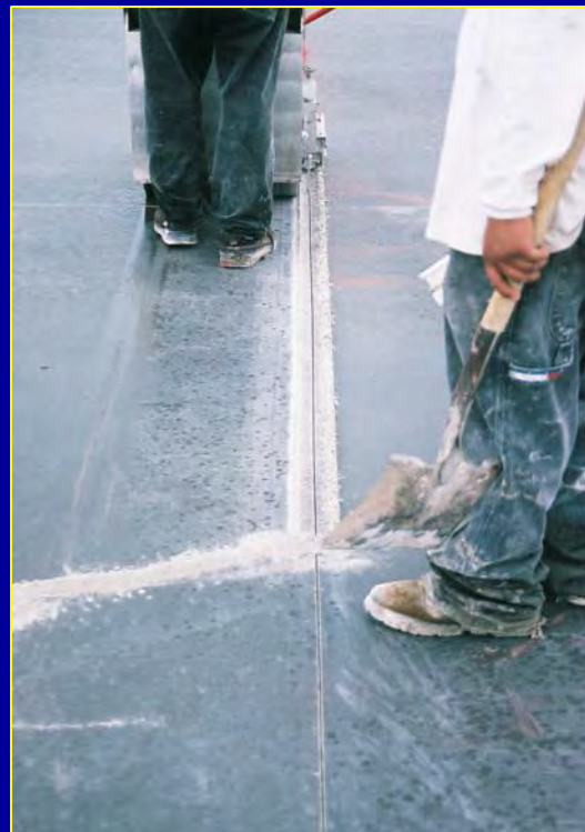
THE FINISHED JOINT
