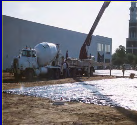
CONCRETE BEING PUMPED
