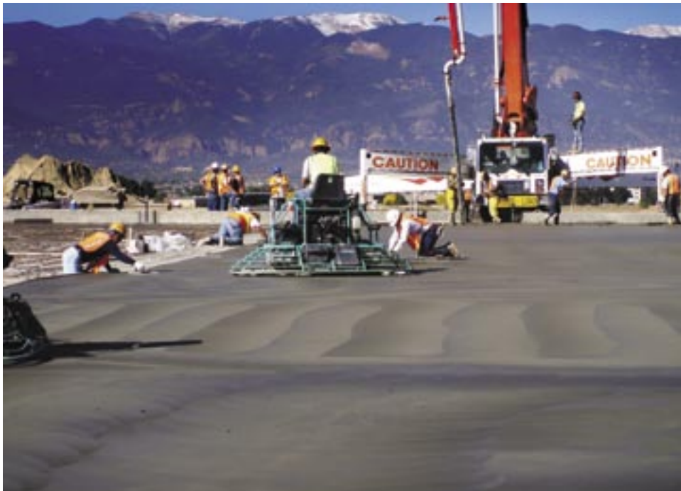
Unsightly balling and fuzz from fibrillated polypropylene
