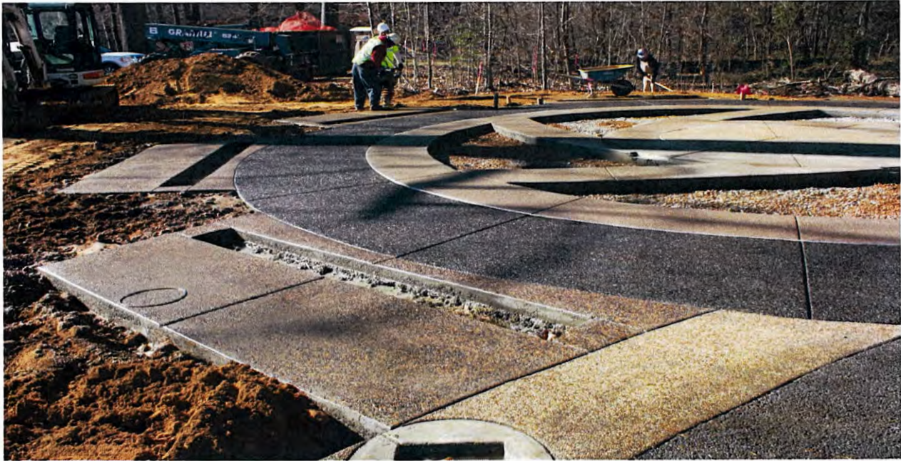
Five different aggregate mixes were employed by Baltz to execute the design, as well as pervious concrete, elements in broom-finish, footers, bollard supports, and notch-bands for donation bricks.
