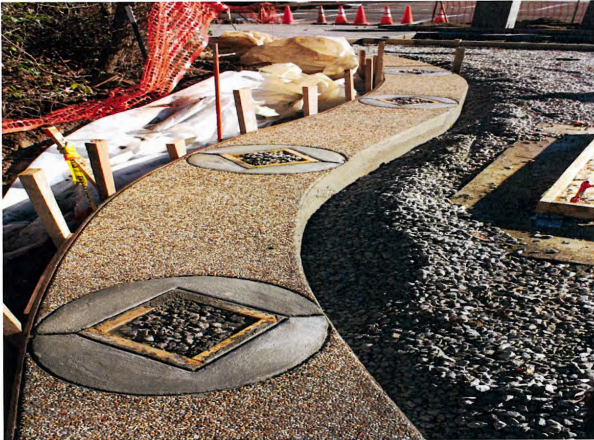
Five different aggregate mixes were employed by Baltz to execute the design, as well as pervious concrete, elements in broom-finish, footers, bollard supports, and notch-bands for donation bricks.
