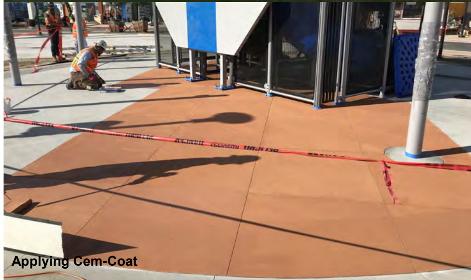
Masking and applying Cem-Coat
